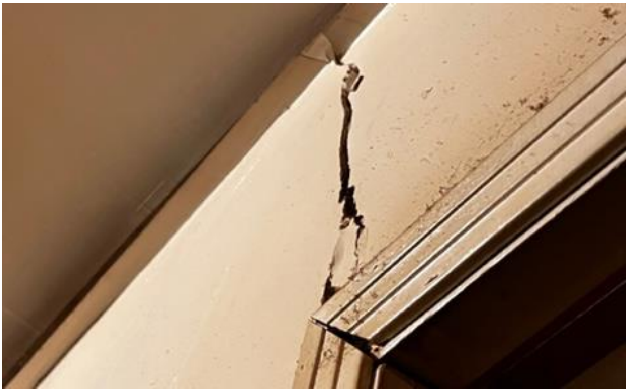
Cracked wall.
