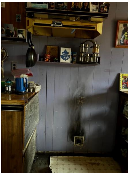
Home without power, water and sanitation. The wiring is a fire hazard and a stove was removed.
